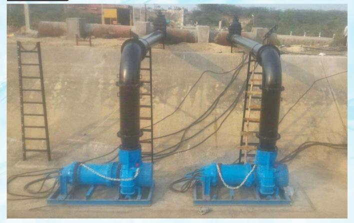
"To eliminate problems associated with earlier p|m; CMC decided to upgrade to Submerged Centrifugal pumpsets (installed directly into Canal - i.e. Flooded Suction).
